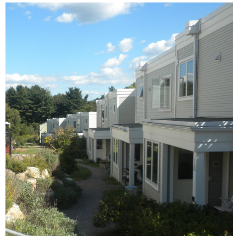
View of green common area, with large community vegetable garden located at the far end of the property.
