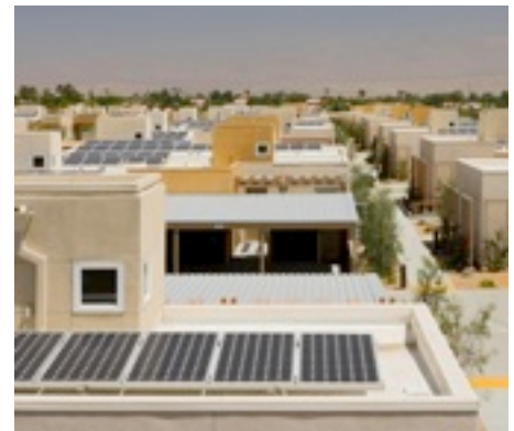
Each unit has a 3 KW photovoltaic system that delivers an average of $730 per year of energy savings.
